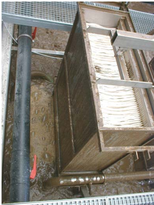
figure 1: Membrane bioreactor system
