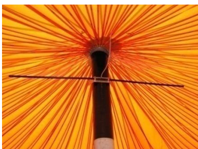
Inside the fermenter – gas storage and desulfurization
