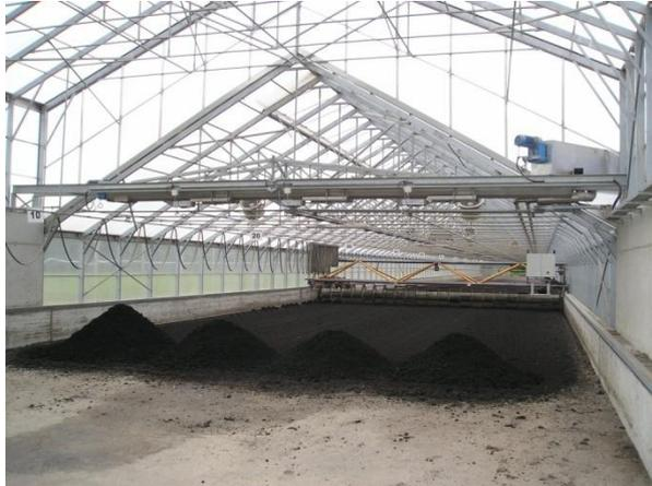
Also the recent adaption of the aerobic purification plant to the state of the art by applying a so-called hybrid process shows a positive effect because a higher amount of sewage sludge and a minor energy demand result from that kind of technology.
