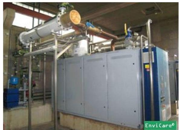
The municipal waste water treatment plant in Knittelfeld has an electrical energy demand of 4.000 kWh/d, which is covered now by its own electricity production in two cogen-units. About 1.900 kWh/d is provided by fermentation of sewage sludge and about 2.100 kWh/d result from fermentation of bio-degradable co-substrates.
