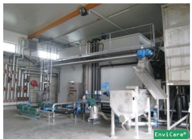
The heat produced in the cogen-unit covers the own requirements completely. Excess heat is supplied for drying sewage sludge.
