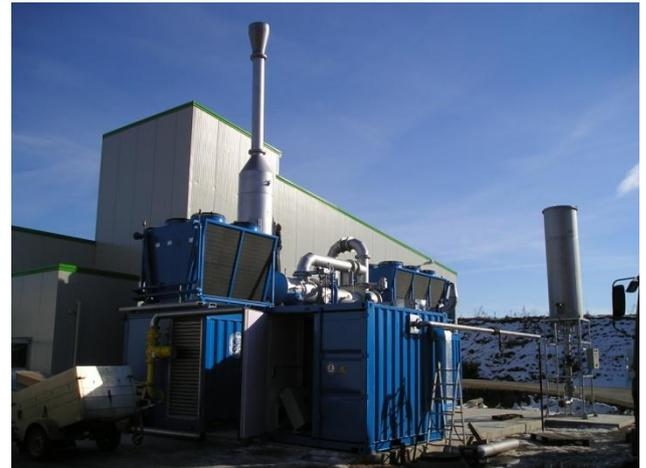
Fig. 6: Combined heat and power station (1.000 kW<sub>el</sub>)
