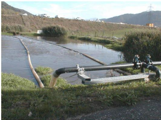
First of all the original wastewater plant, built in 1989 as a ventilated pond purification plant (see left pic.), had to be converted. Two of the three existing lagoons were put out of service, while the remaining lagoon was equipped with an ejector aeration system and a partition wall to create a separate settling basin. In this area sludge is collected and recirculated, the excess sludge is removed with the primary sludge.
