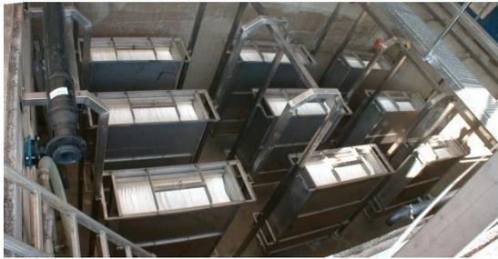
The basin is due to of technical matter constantly aerated by the coarse bubble system.
